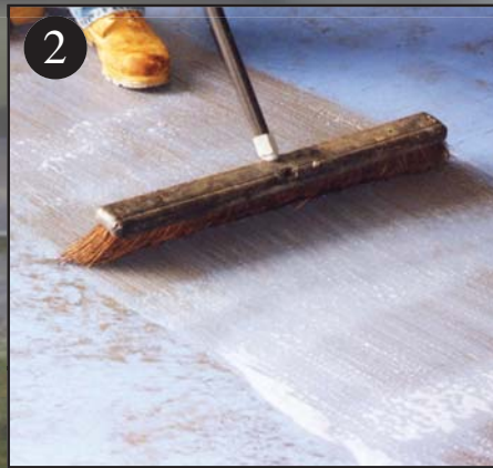
2 Scrub floor with degreaser
