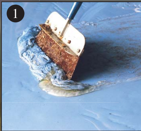
1 Scraping softened epoxy floor paint
