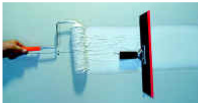
Finish Drywall (Roll on compound, wipe smooth)
