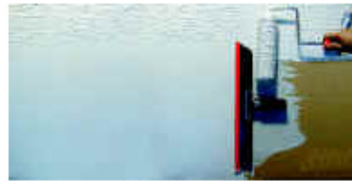
Skimcoat Walls (Roll on like paint, wipe smooth)
